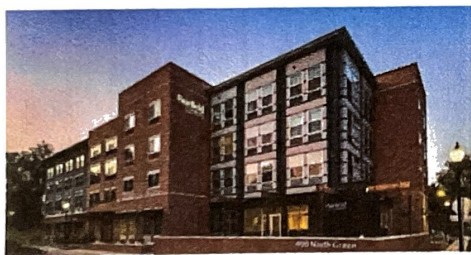
Accommodations Fairfield Inn & Suites 400 North Green St Morganton, NC 28655 844-200-8708
